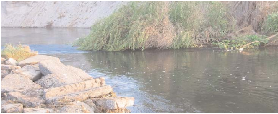
Kings River water flows around a rubble weir near Kingsburg prior to repairs that stabilized a bank that had given way.
