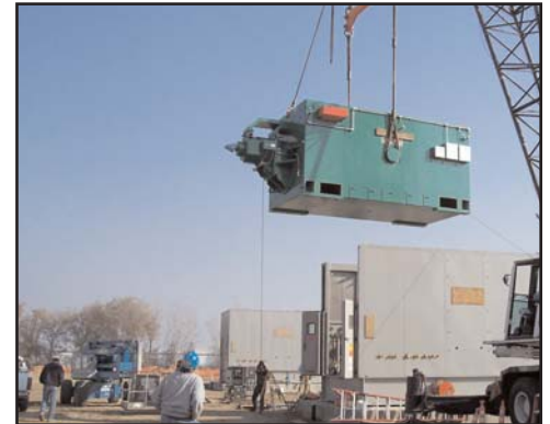
Crews lower one of the generating units into its housing in early December.
