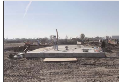
The turbine and generator foundation.
